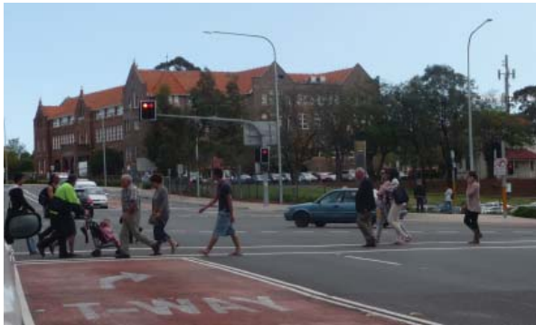
Figure 23. The former St Vincent's Dormitory/School Block on the crest of the hill is visually prominent and forms a terminating vista to Railway Parade.
